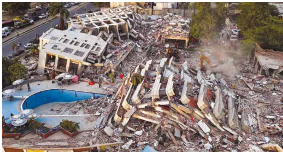
This aerial view shows buildings destroyed following twin earthquakes in Caraballeda, La Guaira State, Venezuela
