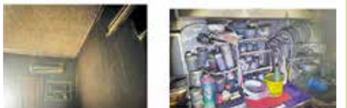
Pictures showing the house fire that displaced a family in A'ali in 2024.
