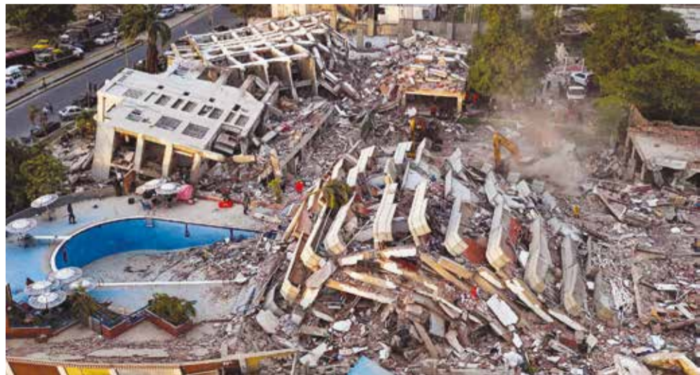
This aerial view shows buildings destroyed following twin earthquakes in Caraballeda, La Guaira State, Venezuela
