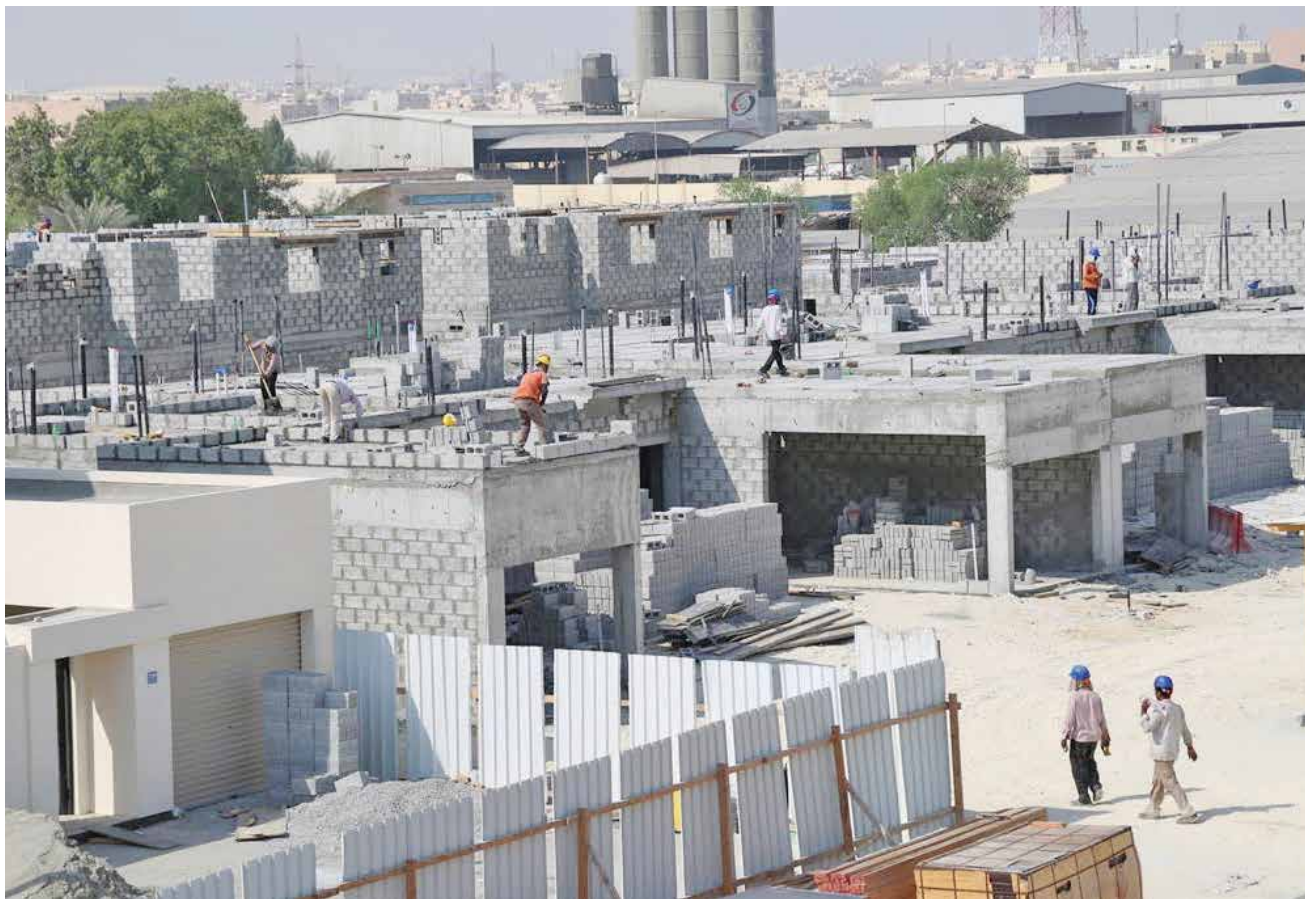
Hawrat Sanad Housing Project third phase in progress
