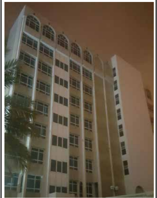
Ministry of Works and Municipalities participated in Earth Hour yesterday by turning off the lights of its buildings and subsidiary projects
