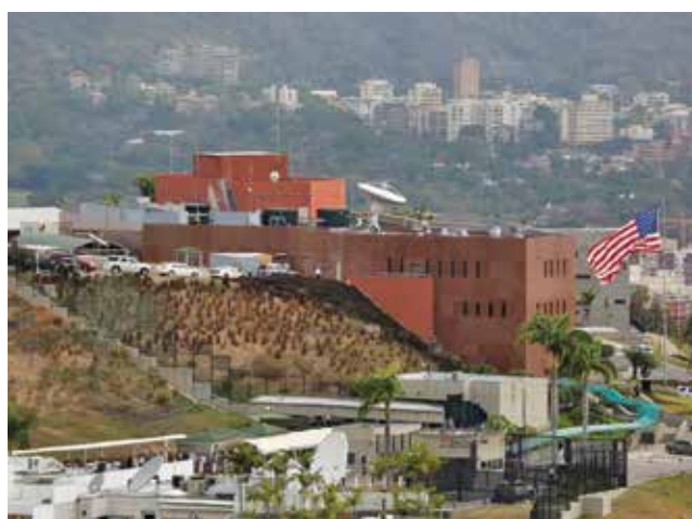
A view shows the U.S. embassy building in Caracas
