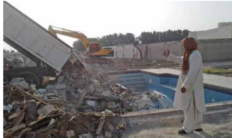
The swimming pool which was demolished by Southern Area Municipality in Dar Kulaib village near Hamad Town
