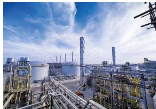
A view shows Saudi Aramco's Wasit Gas Plant (Reuters)
