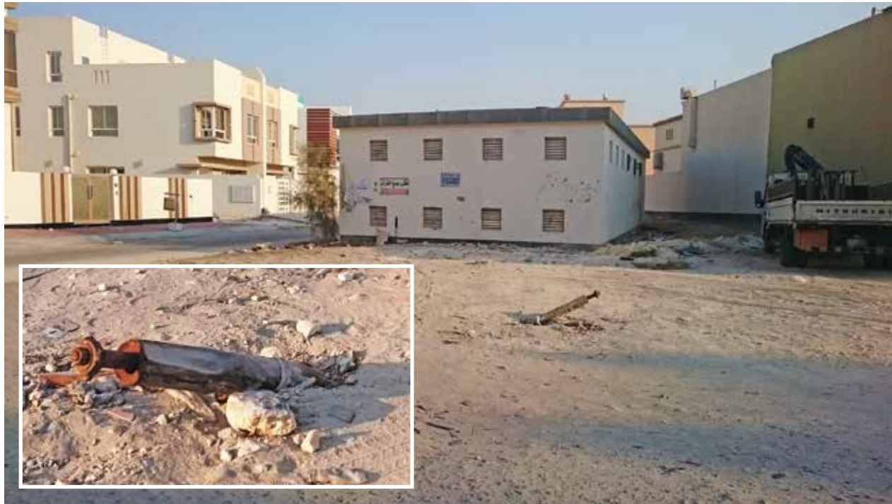
A partially covered cable at a residential area on road no. 724 in Mugaba village, inviting danger as it is usually hit by vehicles. The cable is also posing risk to kids who usually pass through this place.
