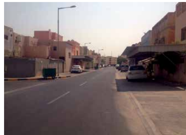
A view of the road included in the project
