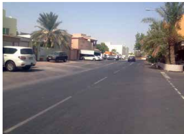
One of the renovated roads.
